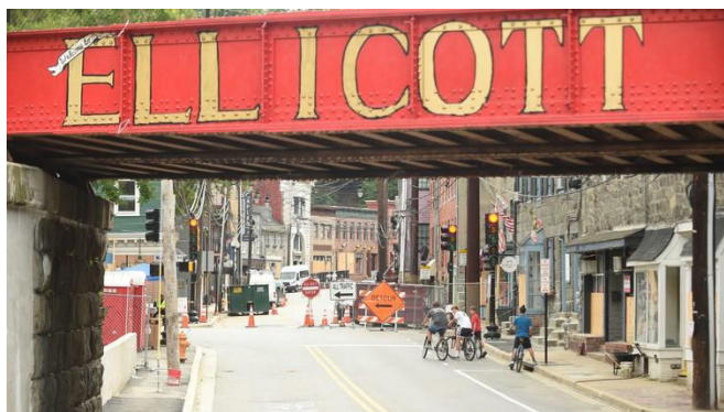
Howard County officials lifted Ellicott City's state of emergency July 20. It was put in place in the aftermath of the May 27 deadly flash flood.
